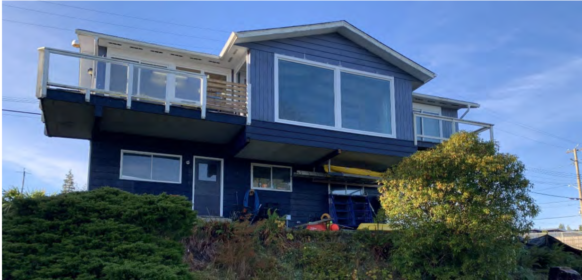
Photo 1. A photo of the back (north) of the house at 1567 Imperial Lane, with the existing deck.
