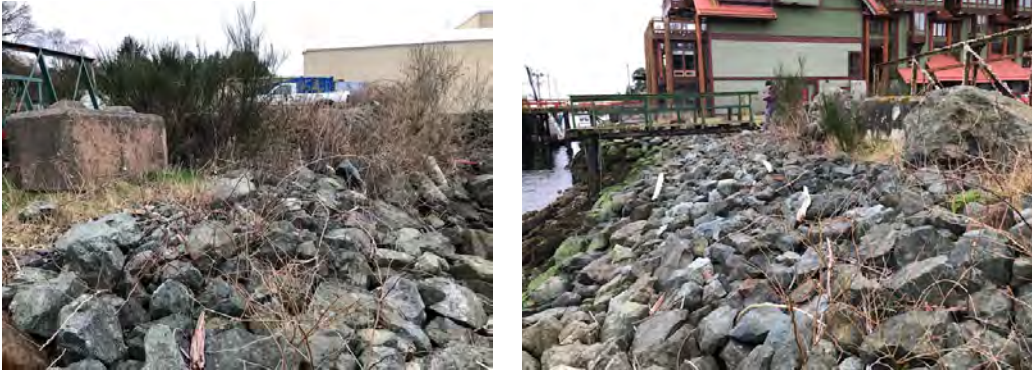
Views north and south along HWM showing upper riprap and riparian zone.
