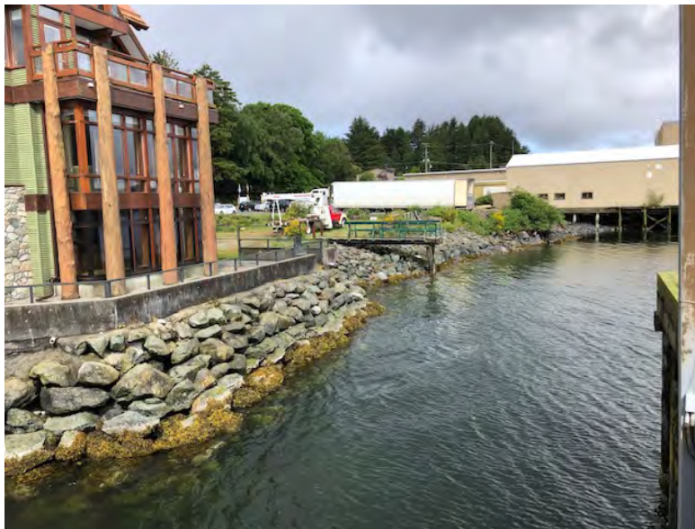
View looking north showing the riprap shoreline at Whiskey Landing Phase I and the vacant lot of Phase II.
