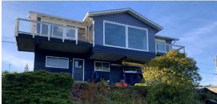
Photo 1. A photo of the back (north) of the house at 1567 Imperial Lane, with the existing deck.
